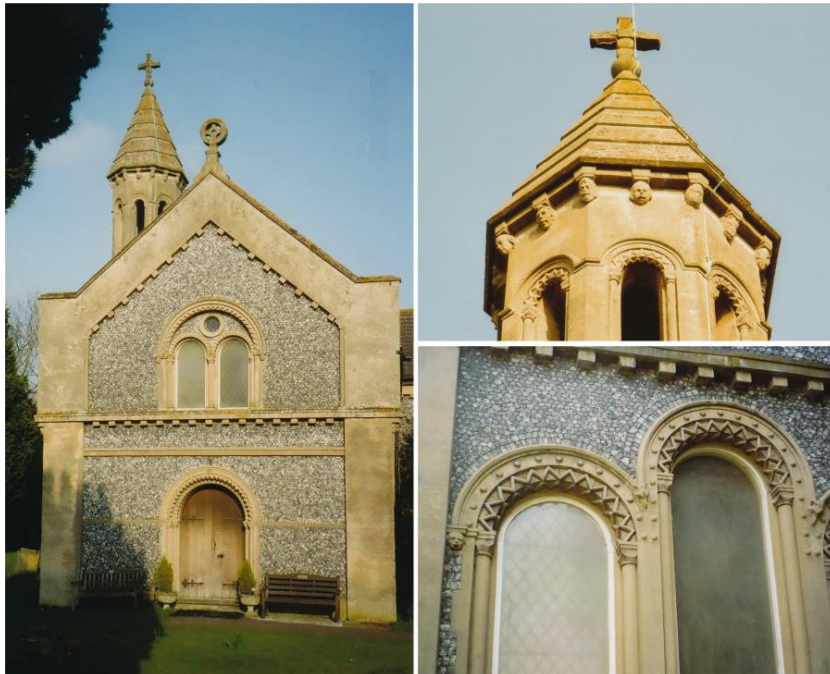
Fig 13 - The knapped flintwork, stone modelling and Pulham faces on the outside of the Church of St Thomas of Canterbury, West Hyde
